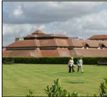
Figure 2: The roof garden on The Willis Building, Ipswich, UK
